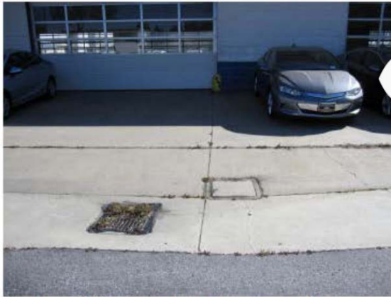
Photograph 23. Concrete access cover (near storm drain at the suspected waste oil UST location at SAC.
